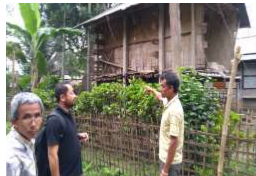
A house damaged by elephant
